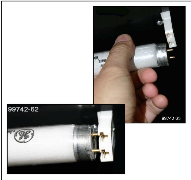
Optional: Lights in Headers Are Accessible From Top of Case. Ample Space is Provided For Lamp Removal/Replacement
